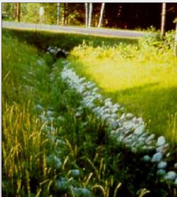
Ditch armored with stone and vegetation
