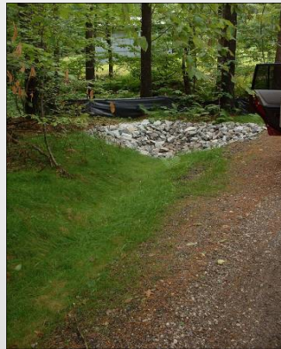
Plunge Pool Collecting runoff
