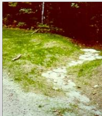
Turnouts direct water into vegetated areas
