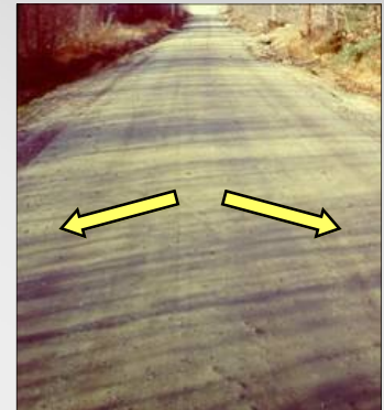
Re-grade Road & add new surface material
