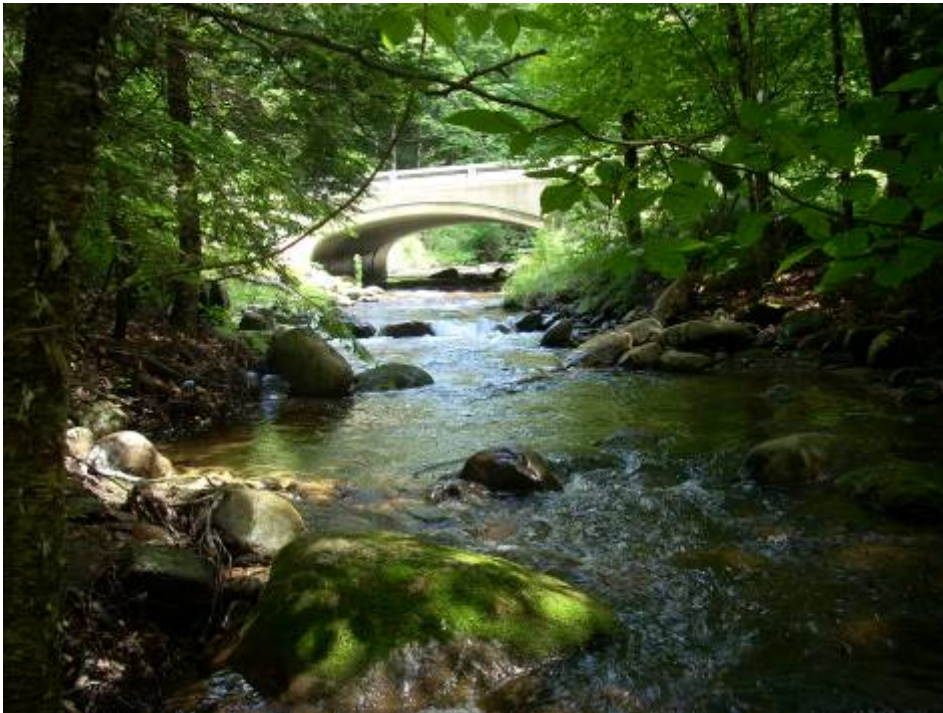
A stream crossing that facilitates fish passage in Belmont (note the natural stream substrate within the stream channel under the crossing). The established riparian buffer seen here also promotes good water quality while providing shade to keep stream temperature cool.
