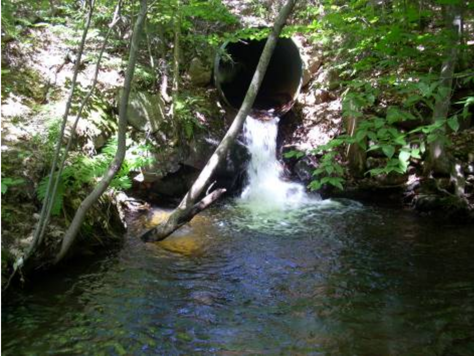
An example of a perched stream crossing in Gilmanston where various fish species may have difficulty accessing essential habitats throughout the year.
