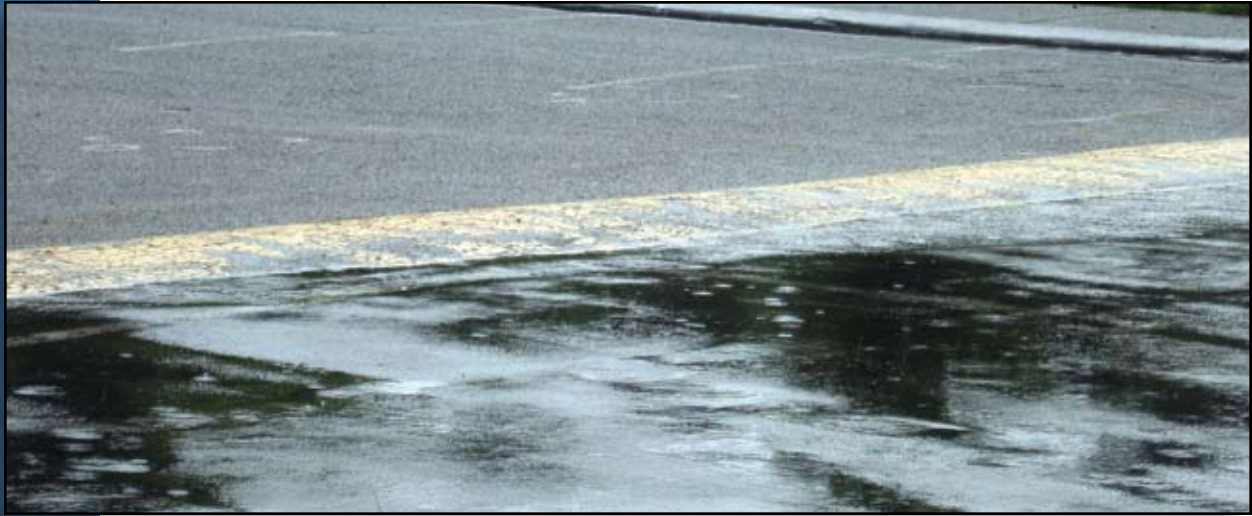
Porous asphalt (top) and dense mix asphalt (bottom) during a heavy rain event.
