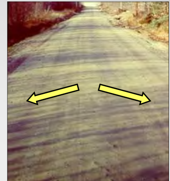
Re-grade Road & add new surface material
