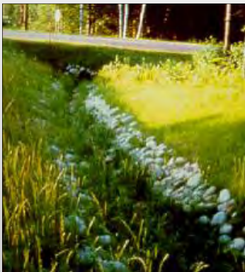
Ditch armored with stone and vegetation
