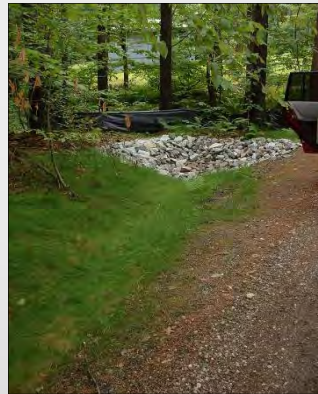
Plunge Pool Collecting runoff
