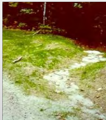
Turnouts direct water into vegetated areas
