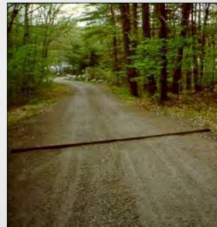
Rubber razors direct water off driveway and into vegetation
