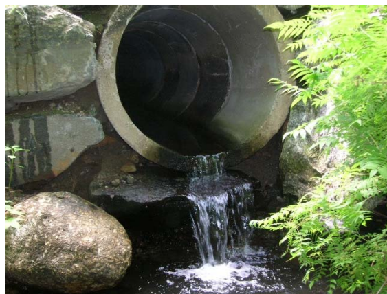
Figure 5. Outlet of perched crossing on Reservoir Rd.
