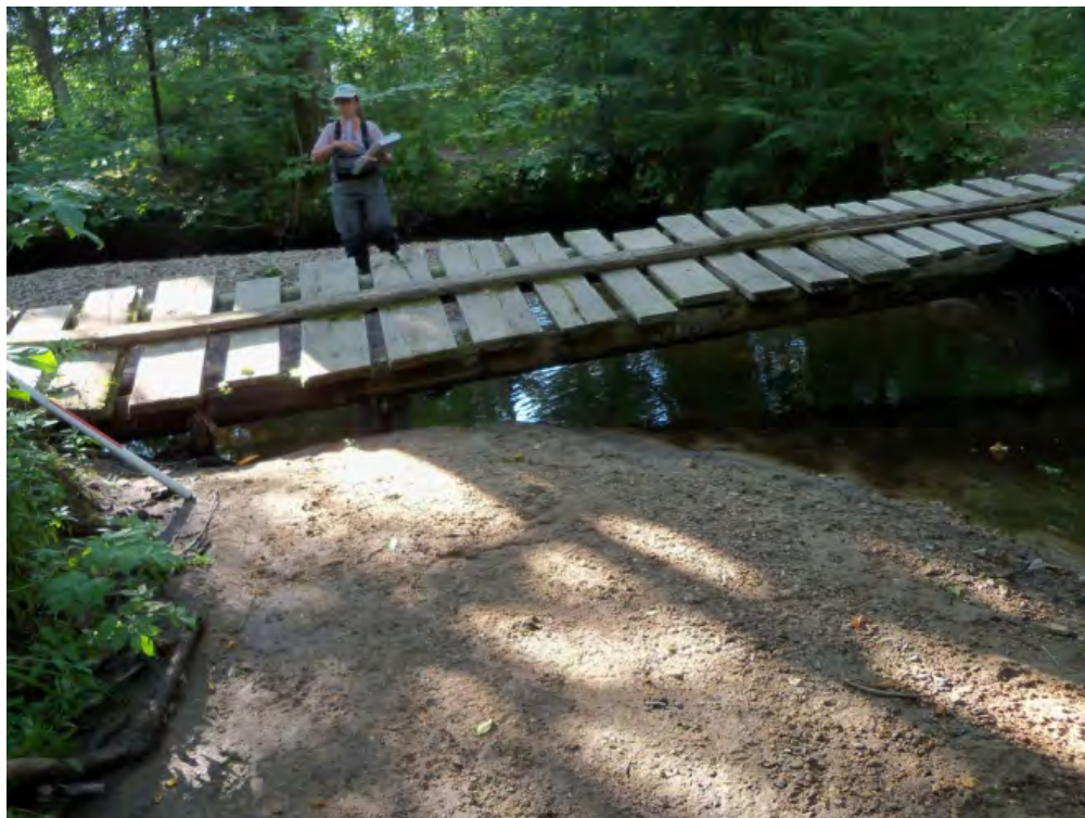
Figure 8.32. Collapsing wooden bridge in M04-B.
