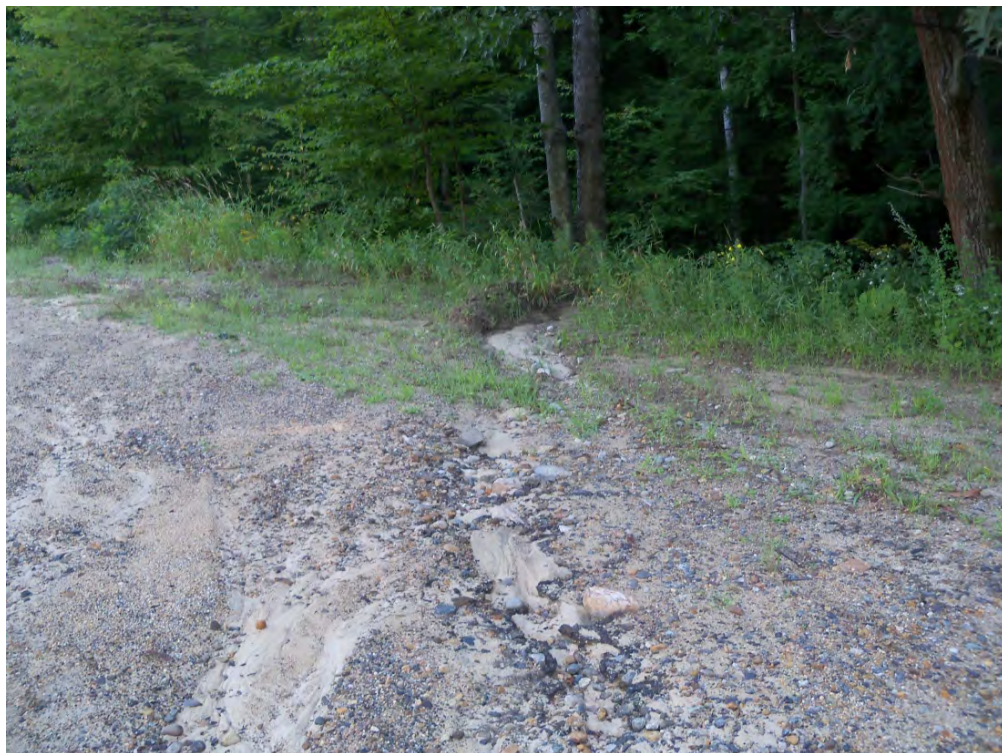
Figure 8.18. Sediment laden stormwater runoff from Town Garage parking lot in M03-A.
