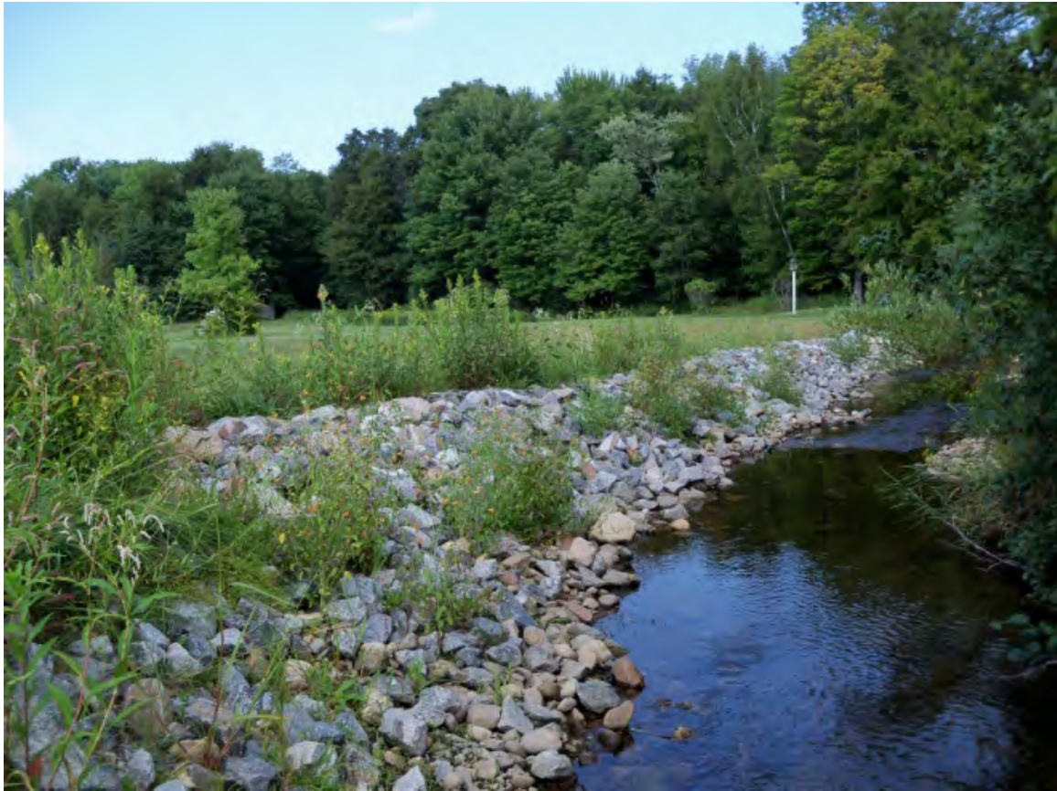
Figure 8.34. Channel alteration and streambank armoring in M04-C.
