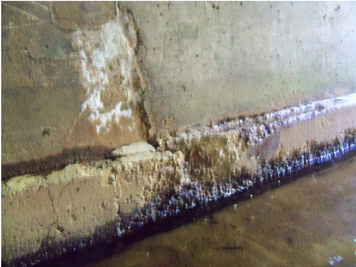
Figure 7.1. The Cherry Valley Road Bridge has deteriorating footers.
