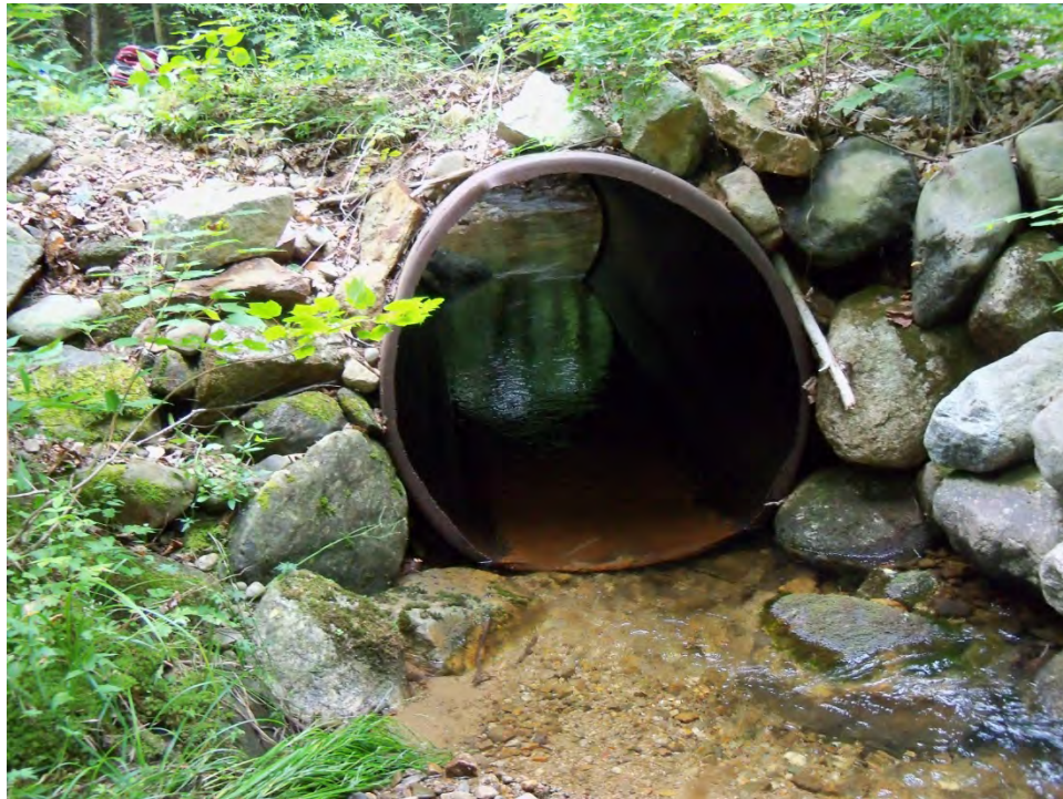
Figure 8.41. Undersized and rusted culvert in T2.01-A.
