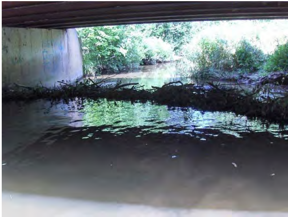
Figure 8.26. Beaver dam within Alvah Wilson Road Bridge in M04-A.
