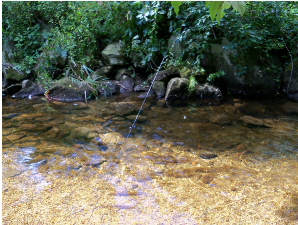
Figure 8.2 Rock riprap in vicinity of measured cross section in M01-B.
