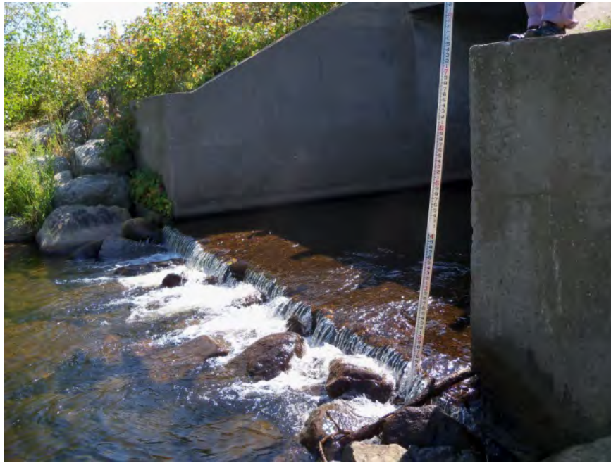
Figure 8.3. Perched box culvert at Lakeshore Road.
