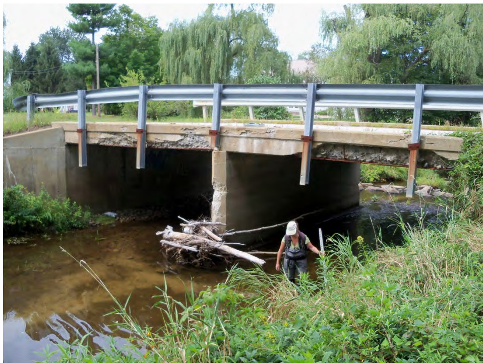
Figure 8.5. Deteriorating decking and pier of Old Lakeshore Road Bridge in Segment M01-B.
