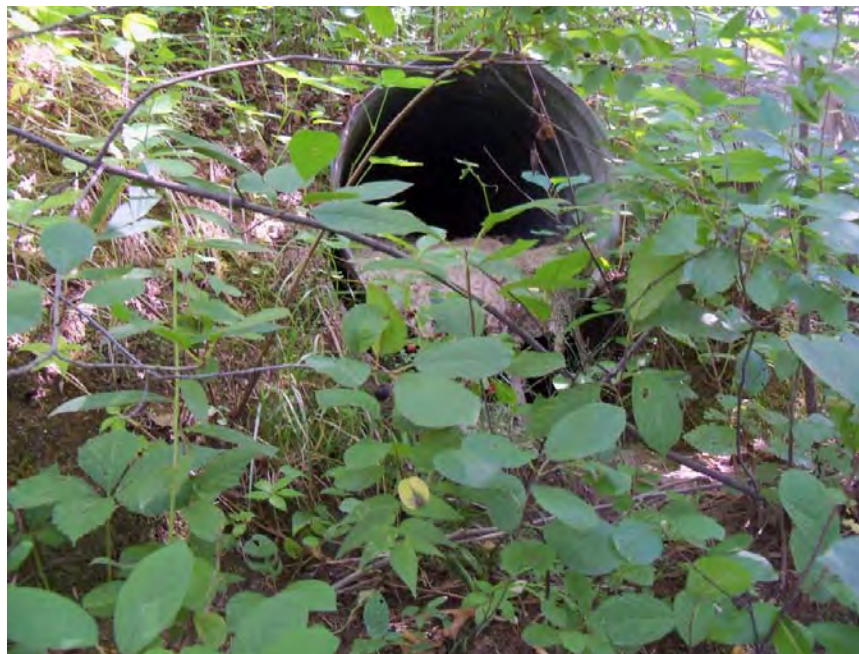
Figure 8.4 Sediment laden stormwater culvert along segment M01-B.
