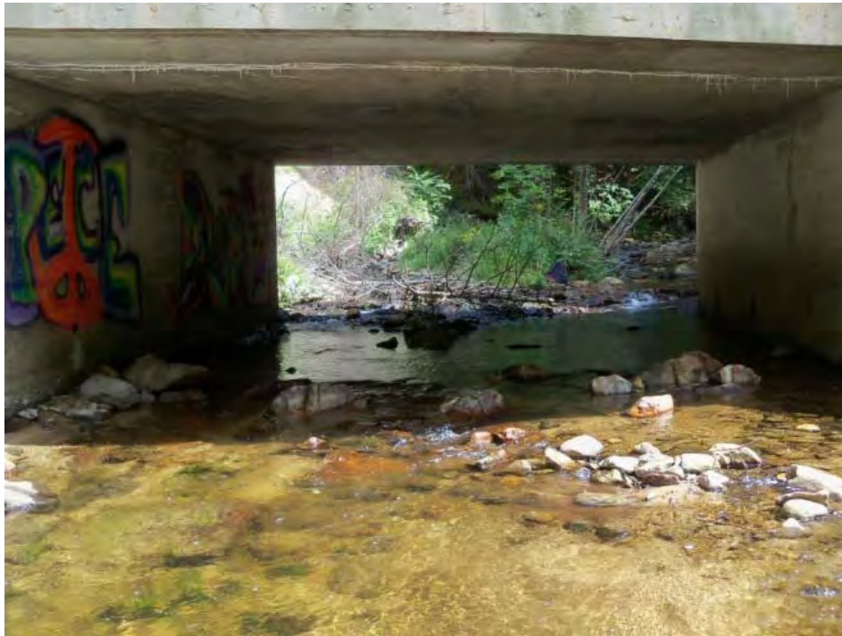
Figure 8.10. Undersized and misaligned Intervale Road Bridge with mid-channel bar upstream in M02-A.
