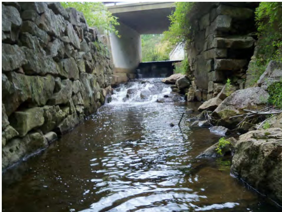
Figure 8.23. Rock walls downstream of the Belknap Mountain Road crossing in M03-B.
