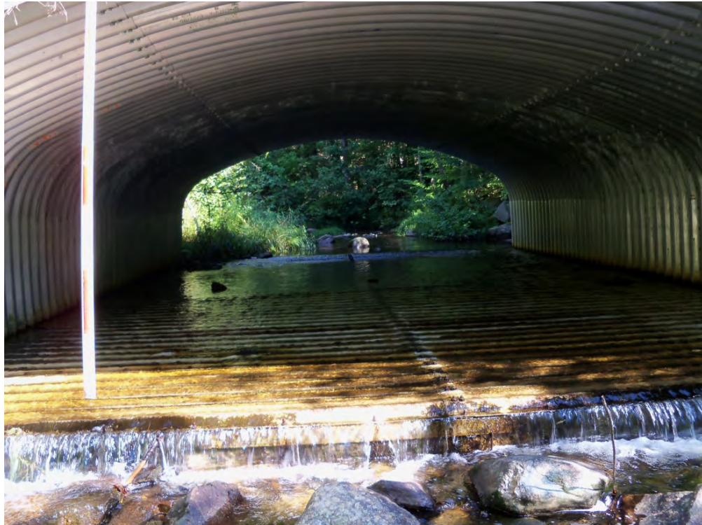
Figure 8.17. Perched culvert at Town Garage Access Road in Segment M03-A impeding aquatic organism passage.
