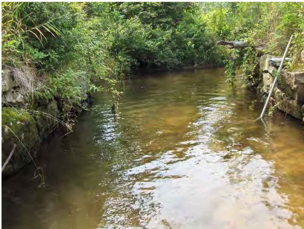
Figure 8.27. Old abutment constricting the stream channel in M04-A.
